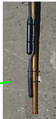
Fixed to the Aquatrak Sounding tube
